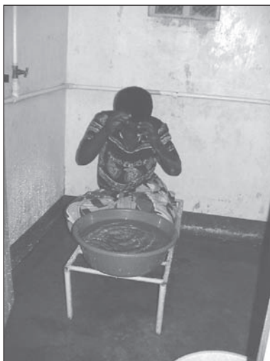
Figure 9.99. Bathroom with room for bathing bench and wheelchair beside it. Tap is within reach of bather.
