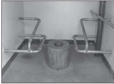
Figure 9.124. Raised toilet seat with handrails for support.
