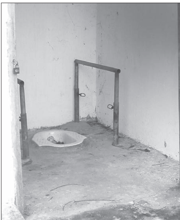
Figure 7.17. Handrails of adjustable height, suitable for a growing child. (Case-study 9.16, page 207)
