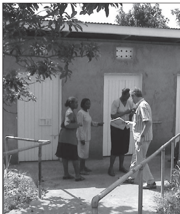
Figure 5.10. Wide concrete ramp with handrails both sides.
