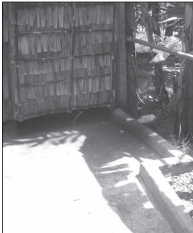
Figure 9.71. Flat platform in front of toilet door.
