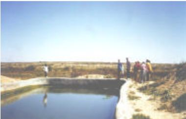
An existing berkad in Hedinta. Note the exposed surface (cause), which may lead to high evaporation and poor bacteriological quality (symptom).
