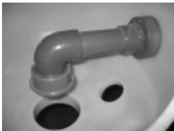
5.- Glue the piping necessary to adapt accessories and screw required arms to the distributor to complete the distribution system.
