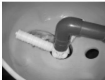
5.- Glue the piping necessary to adapt accessories and screw required arms to the distributor to complete the distribution system.
