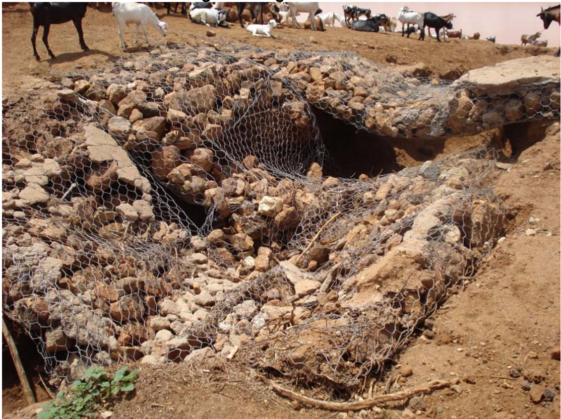
Photo 22b: Gabions damaged during floods
