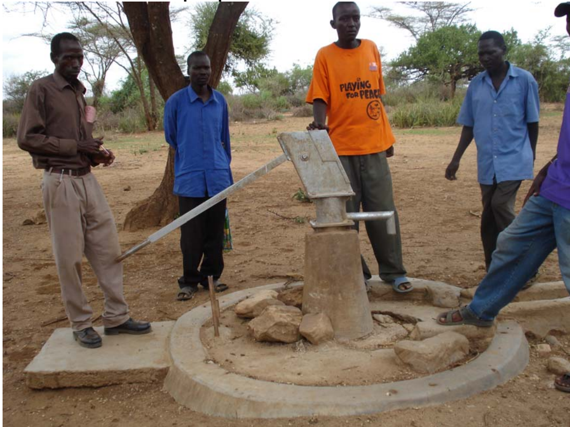
Photo 17: Broken handpump
