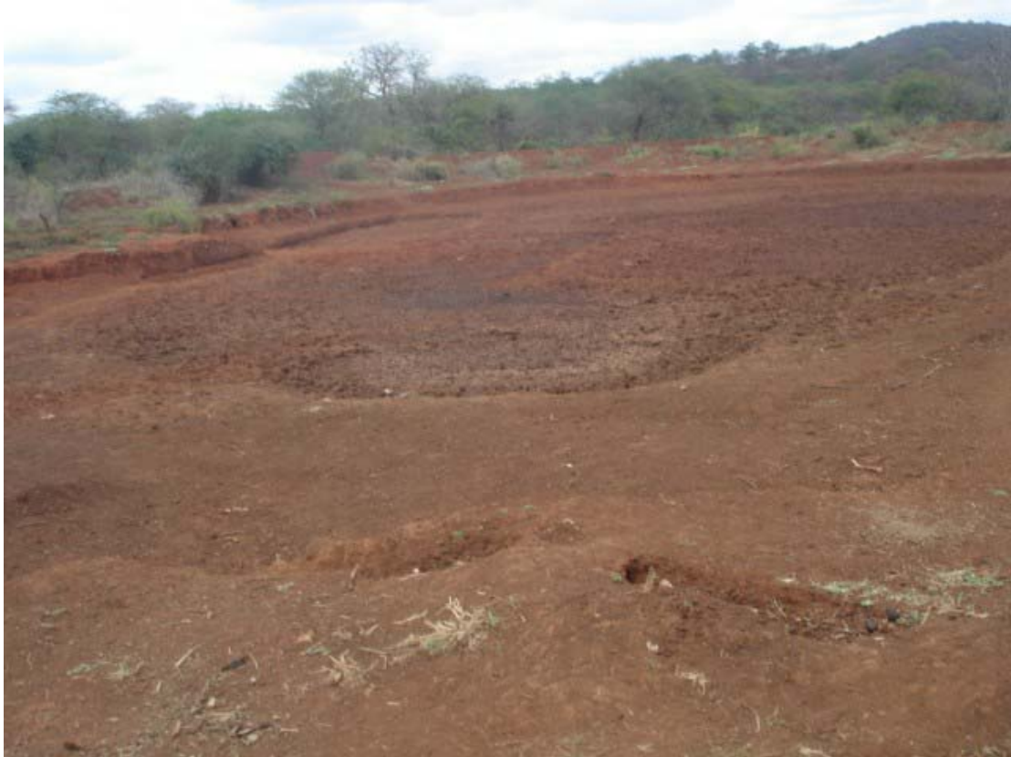
Photo 23: Water Pan silted
