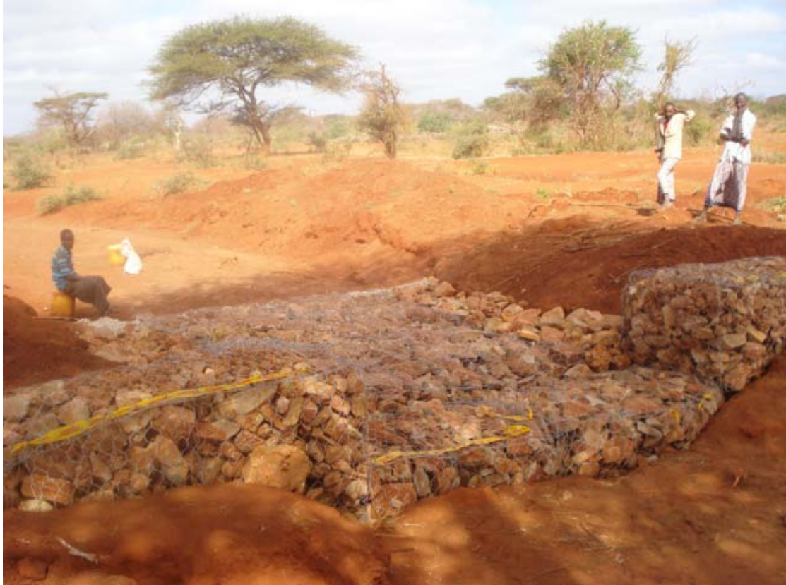
Photo 22a: Newly laid inlet using gabions and rip-rap
