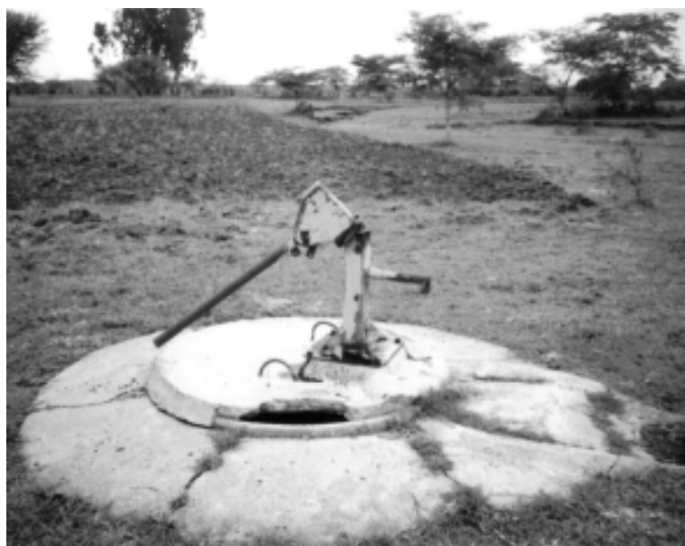
Lack of a sense of communal ownership left many of the installed water systems in poor state as shown in this picture of an abandoned well with a broken hand pump in one of the villages in Shinyanga District.
