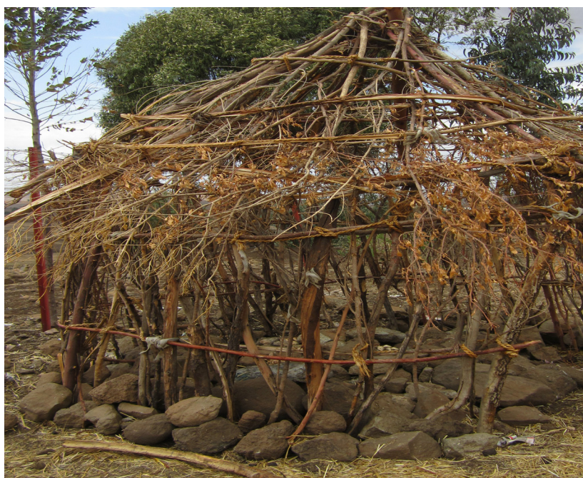
Partially constructed household latrine in Senbetge, North Gondar, made from locally available materials.
