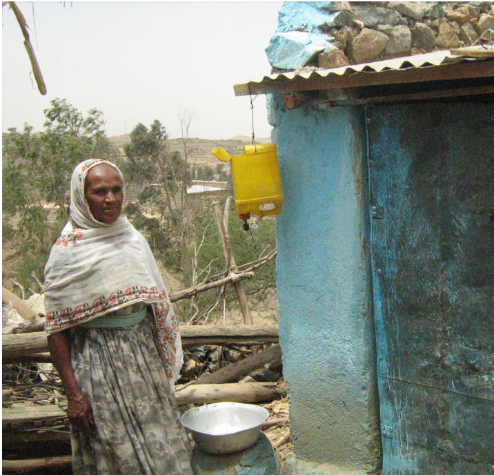
Household latrine in Eritrea, with locally made hand-washing facilities using a jerry-can.
