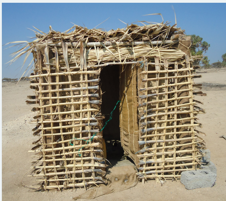
Household latrine in the lowlands of Eritrea, made from locally available materials as part of the CLTS/PHAST process implemented under RCSE's RWSP.
