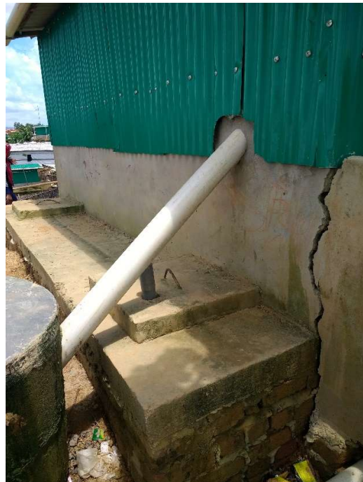
PVC pipe connecting inside of latrine to a sealed pit for collecting menstrual waste, in Camp 19.
