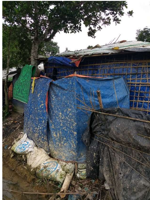
Informal/unplanned bathing area constructed off the back of a shelter in Camp 19. Main materials used are bamboo, tarpaulins and sandbags.
