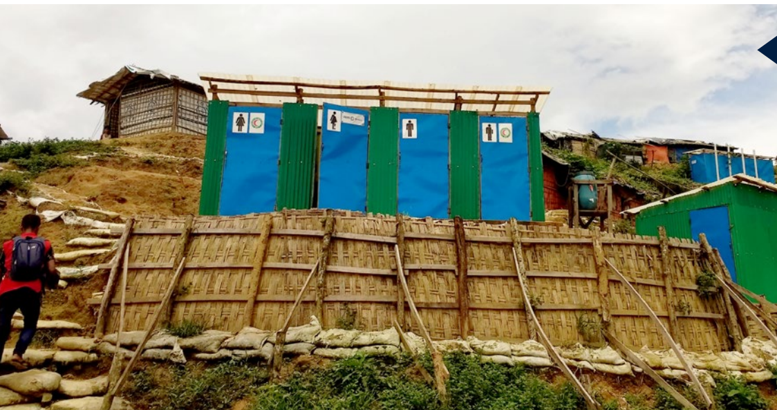
Block of latrines in Cox's Bazar
