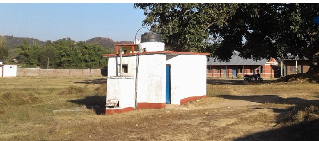
Gender friendly school toilet with incinerator for menstrual waste, Dang.
