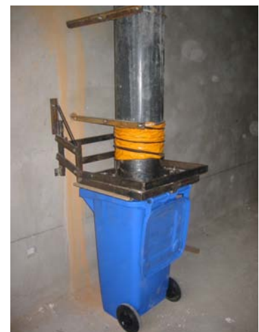
Figure 4-13: Straight-drop dry urine-diverting toilet in multi-story apartments in Dong Sheng, Inner Mongolia, Northern China including illustrations of the porcelain toilet and fecal bin (SEI)
