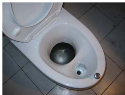
Figure 4-13: Straight-drop dry urine-diverting toilet in multi-story apartments in Dong Sheng, Inner Mongolia, Northern China including illustrations of the porcelain toilet and fecal bin (SEI)
