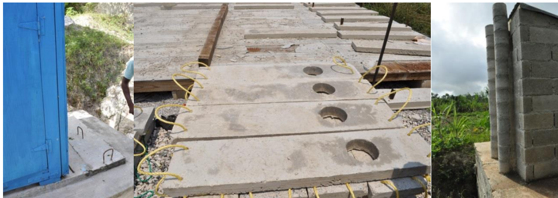
Picture series 7 L to R – Norwegians RC Petit Goave slab - rebar handles/ties, Swiss Leogane slab – nylon rope handles, Netherlands- Leogane removable slabs.
