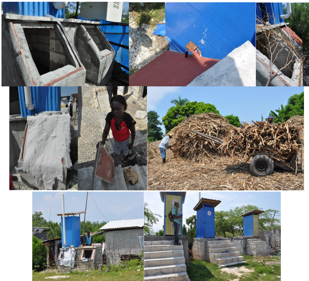
Picture Series 12: IFRC Leogane Bagadere area Eco Latrines. Top Row L to R: Missing hatches, locked hatched and sticker bushes covering hatch. Middle Row L to R: Latrine in use with cloth cover over hatch hole, woman showing hatch from slab she was keeping inside her home and sugar cane stalk collection point. Bottom Row L to R: latrines (three on the right were not being used)
