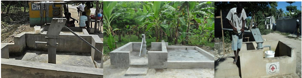
Picture Series 5 Borehole wells - GRC/AutRC - Leogane borehole wells with India Mark II handpumps; IFRC – Tamarin New Drilled Borehole
