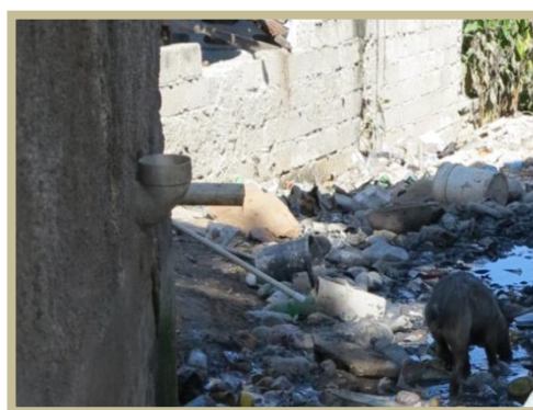
Photo CFF_4: Toilet discharge to canal
