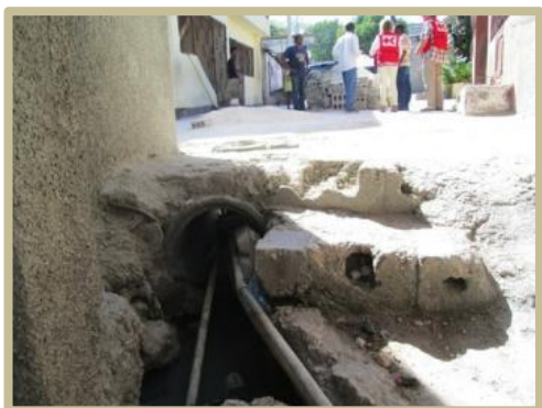
Photo D911_1: Water pipes inside drainage
