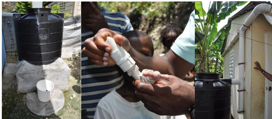
Picture series 2 HH Rain Catchment systems L to R: Norwegian RC-Petit Goave system anchored in concrete, with concrete skirt, an example of a broken tap, PVC piping securely anchored to the house with first flush outtake valve.
