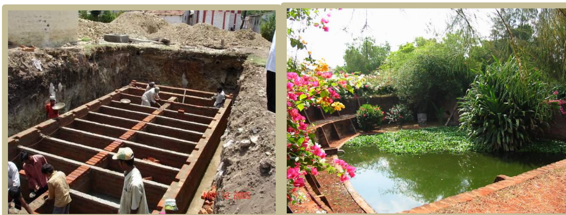
Figure 2: Left - DEWATS baffled reactor under construction; Right -DEWATS polishing pond
