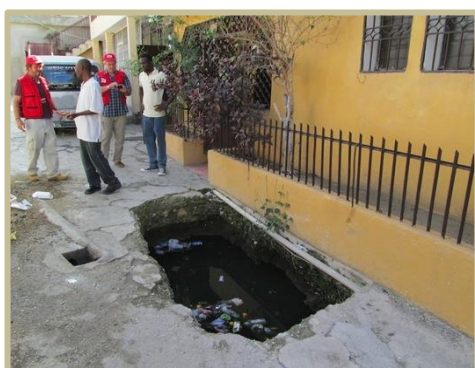
Photo D30_1: Collapsed septic tank
