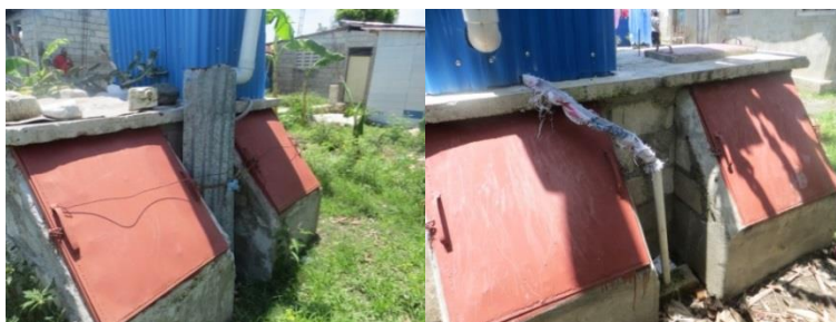
Picture Series 11 IFRC Leogane Neply EcoSan Latrines. (Note locking system and HH added support/protection for the urine diversion pipes)
