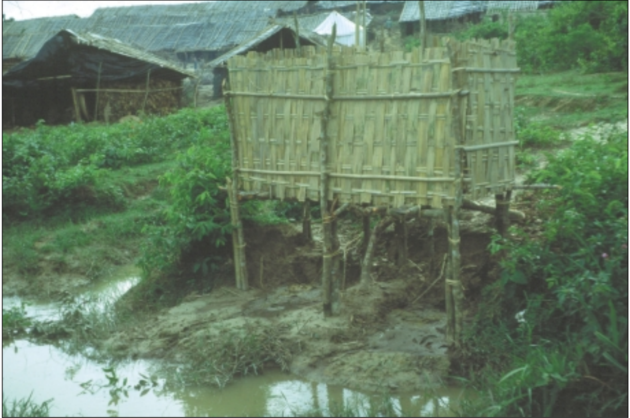
Overhung latrine, Bangladesh
