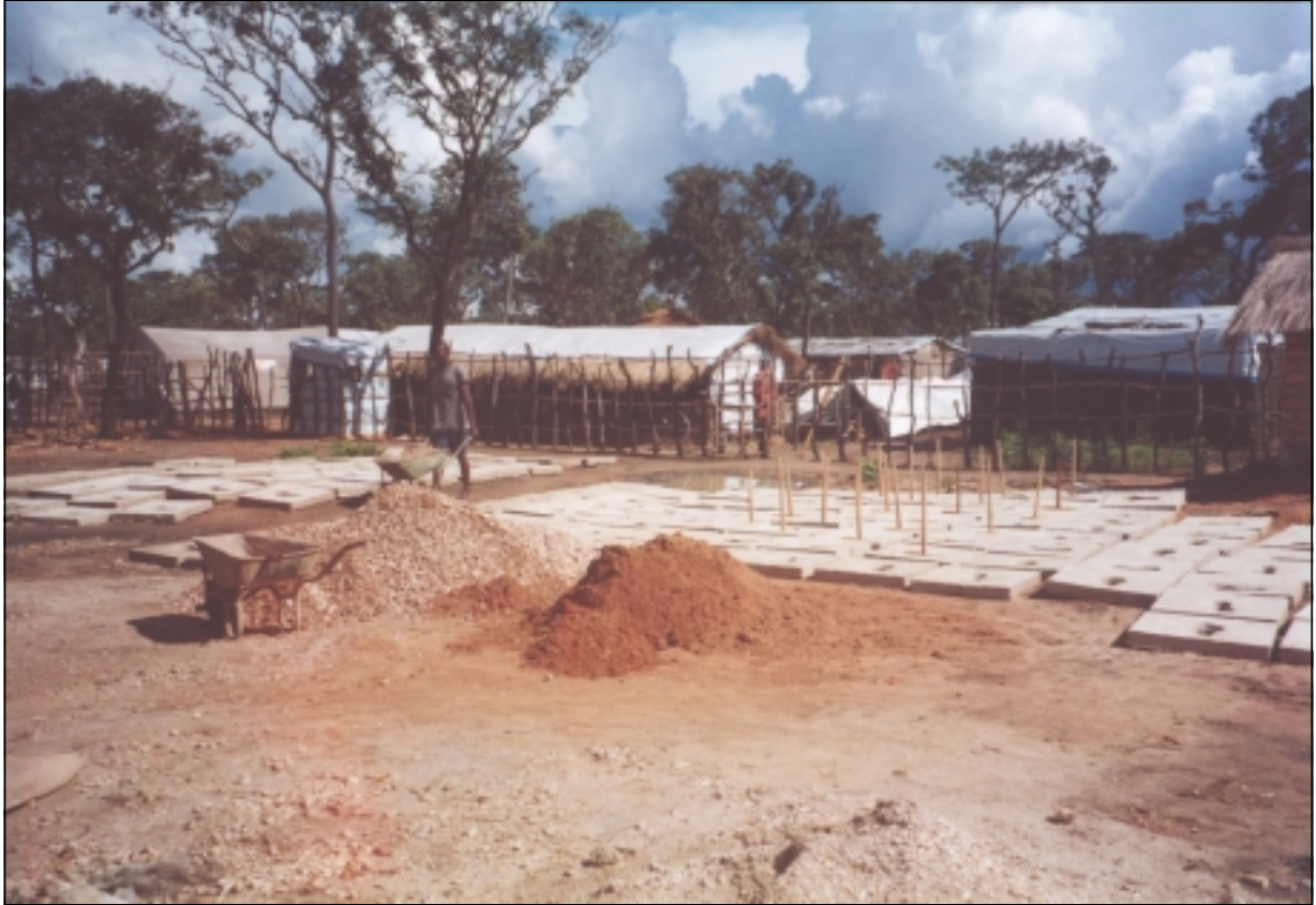
Preparation of concrete latrine slabs
