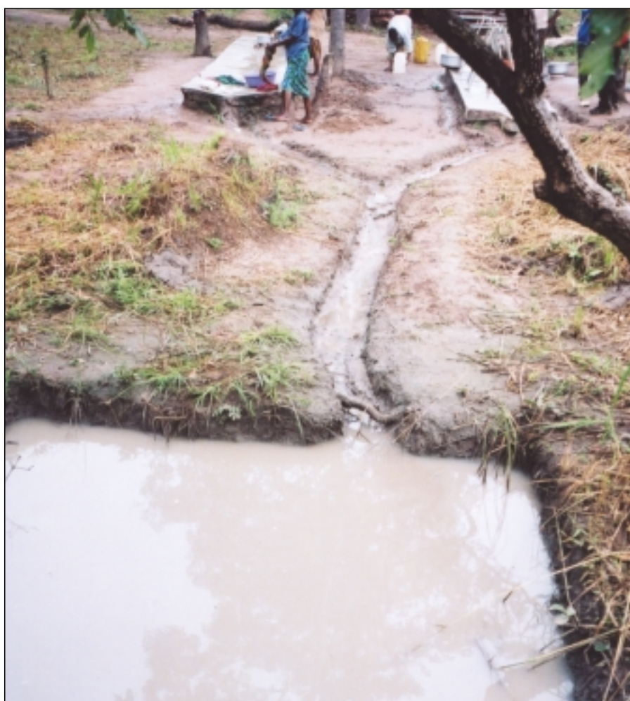
Poorly designed soakpit, Tanzania
