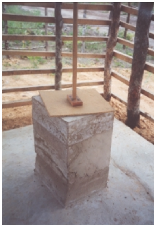
Sealed sharps pit, Zambia
