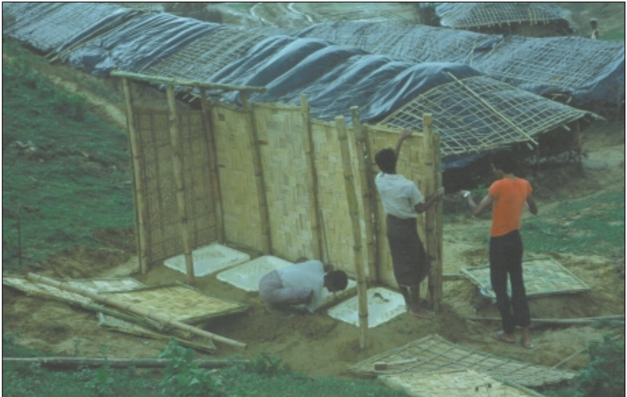
Borehole latrines nearing completion, Bangladesh
