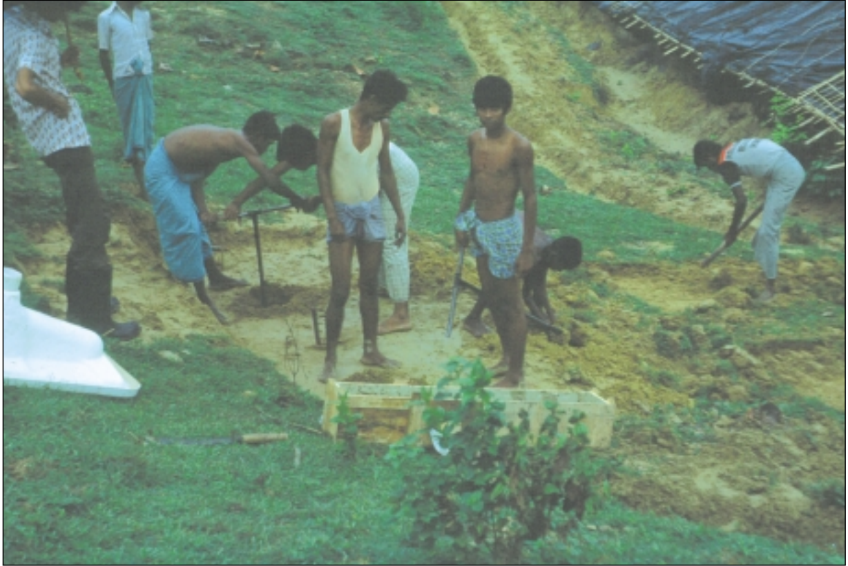
Drilling boreholes for latrines, Bangladesh
