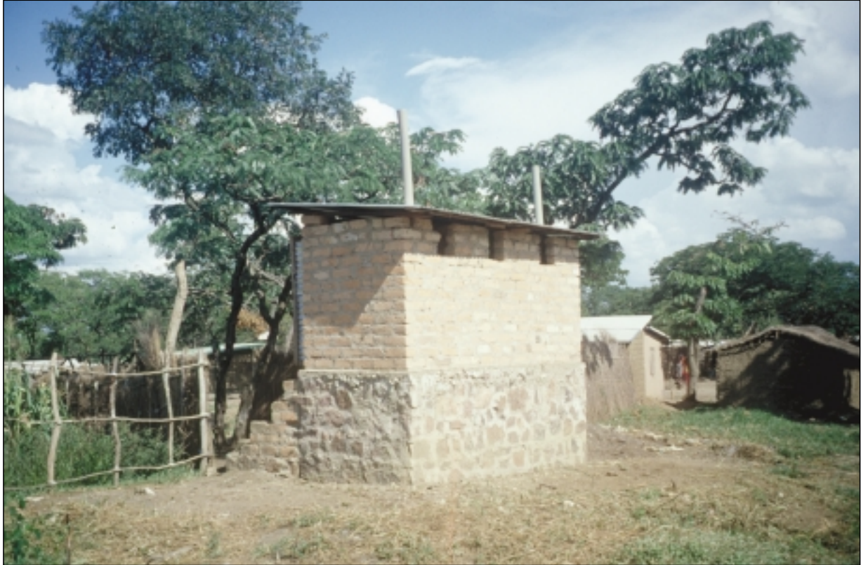
Raised VIP latrines, Tanzania
