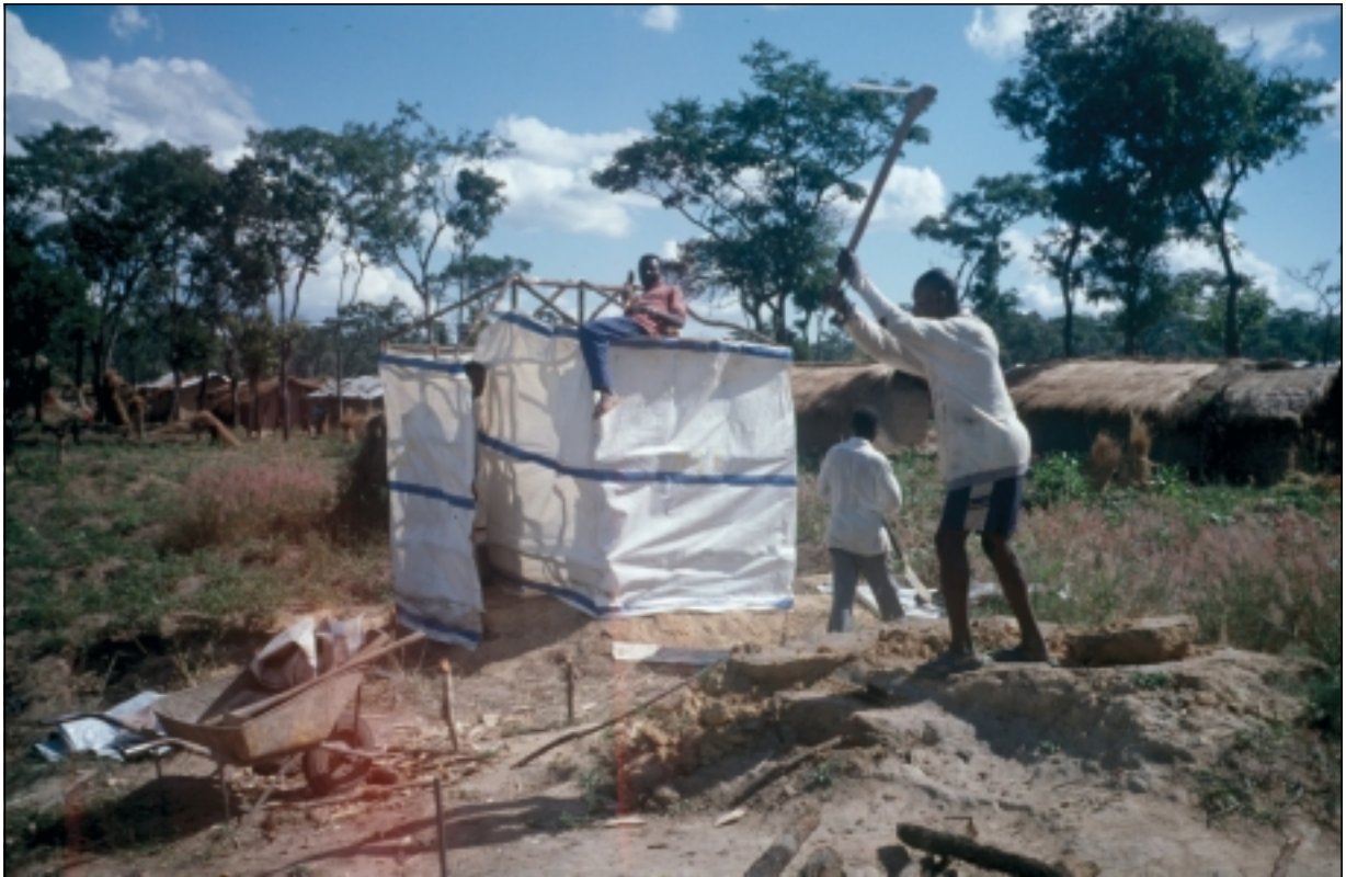
Pit latrine construction
