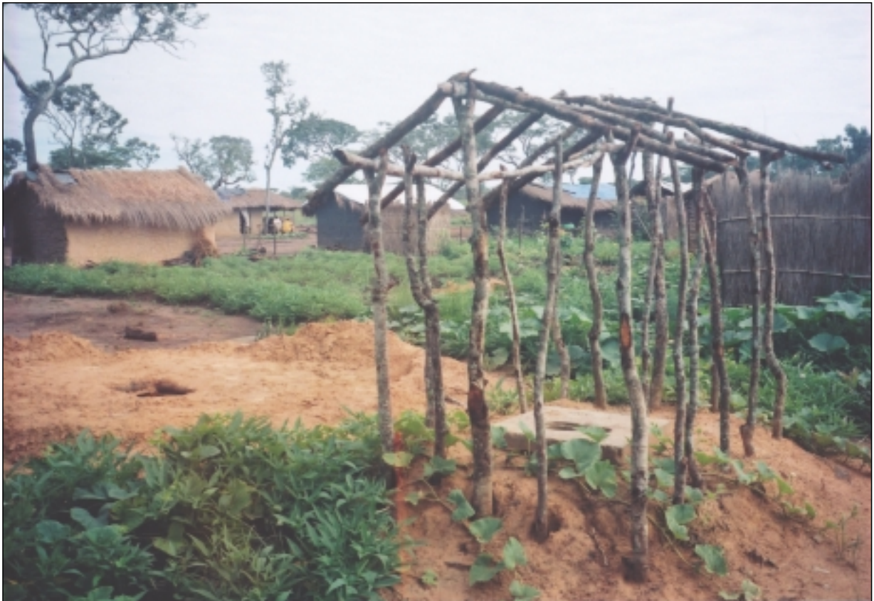
Family pit latrine under construction
