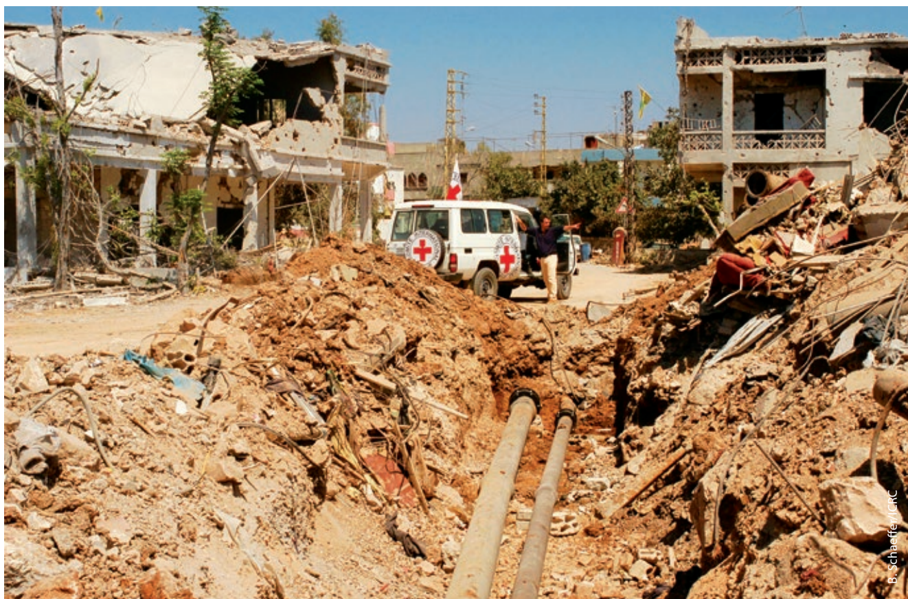
Photo 3. Direct and indirect impact starting to accumulate. It may be possible to repair these pipes but if water pressure remains insufficient, local residents are likely to install suction pumps – a “negative” coping mechanism that places the health of many more people at risk. (Southern Lebanon, 2006)
