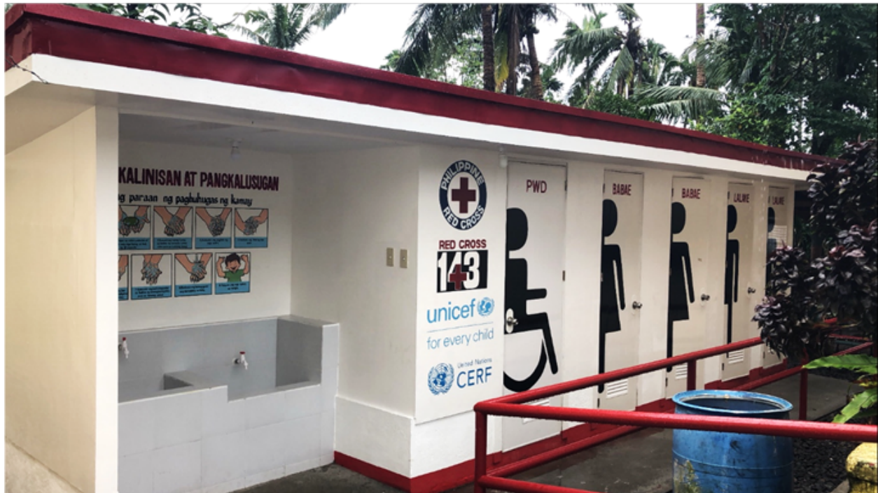
5-seater transitional toilets with PWD room, locks, ramps and railings San Roque Evacuation Center, Malilipot, Albay.
